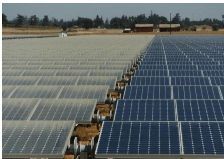
Figure 1.1.1: Aerial view of a solar farm highlighting clean vs. dirty panels
