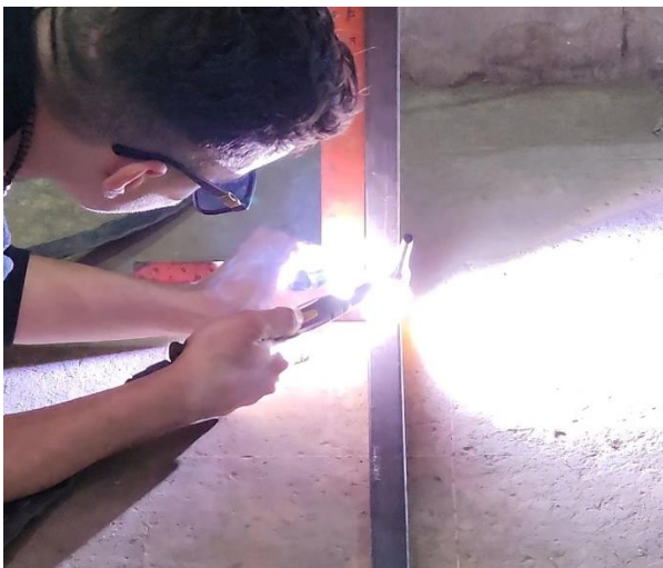
Figure 2.6.2: Welding using Argon technique
